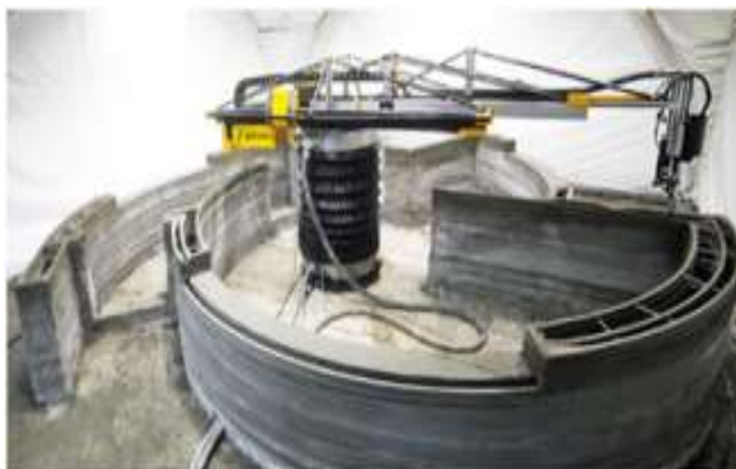
Pic. 3. Printer with a telescopic device
